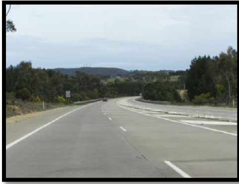
(a) paver block road
